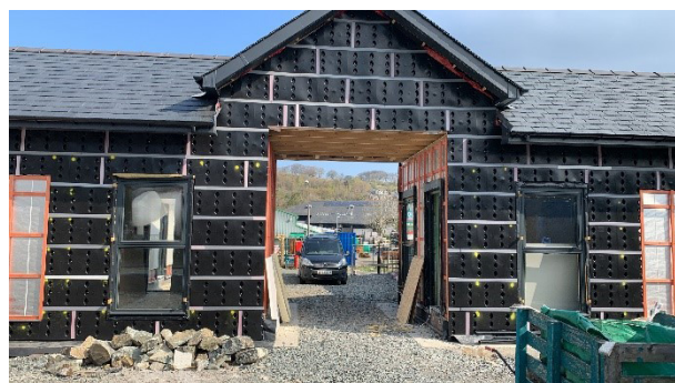
The former Ysgol Glan Wnion is about to receive a new stone face.
